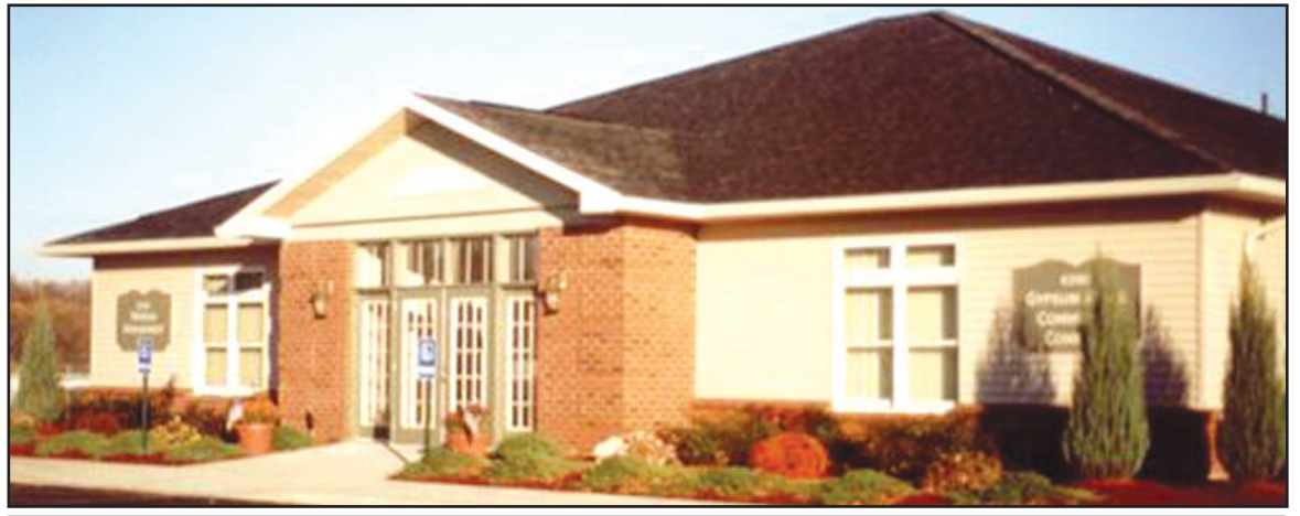
Gypsum Mills Mobile Home Community, Victor
